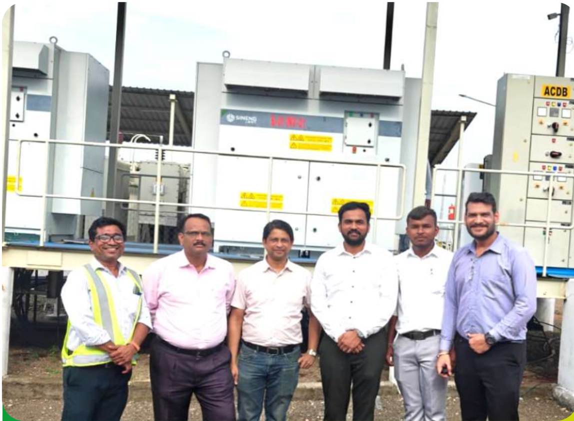
Successful Charging of the 25 MW Solar Power Plant with Mahagenco, Godrej & Boyce
