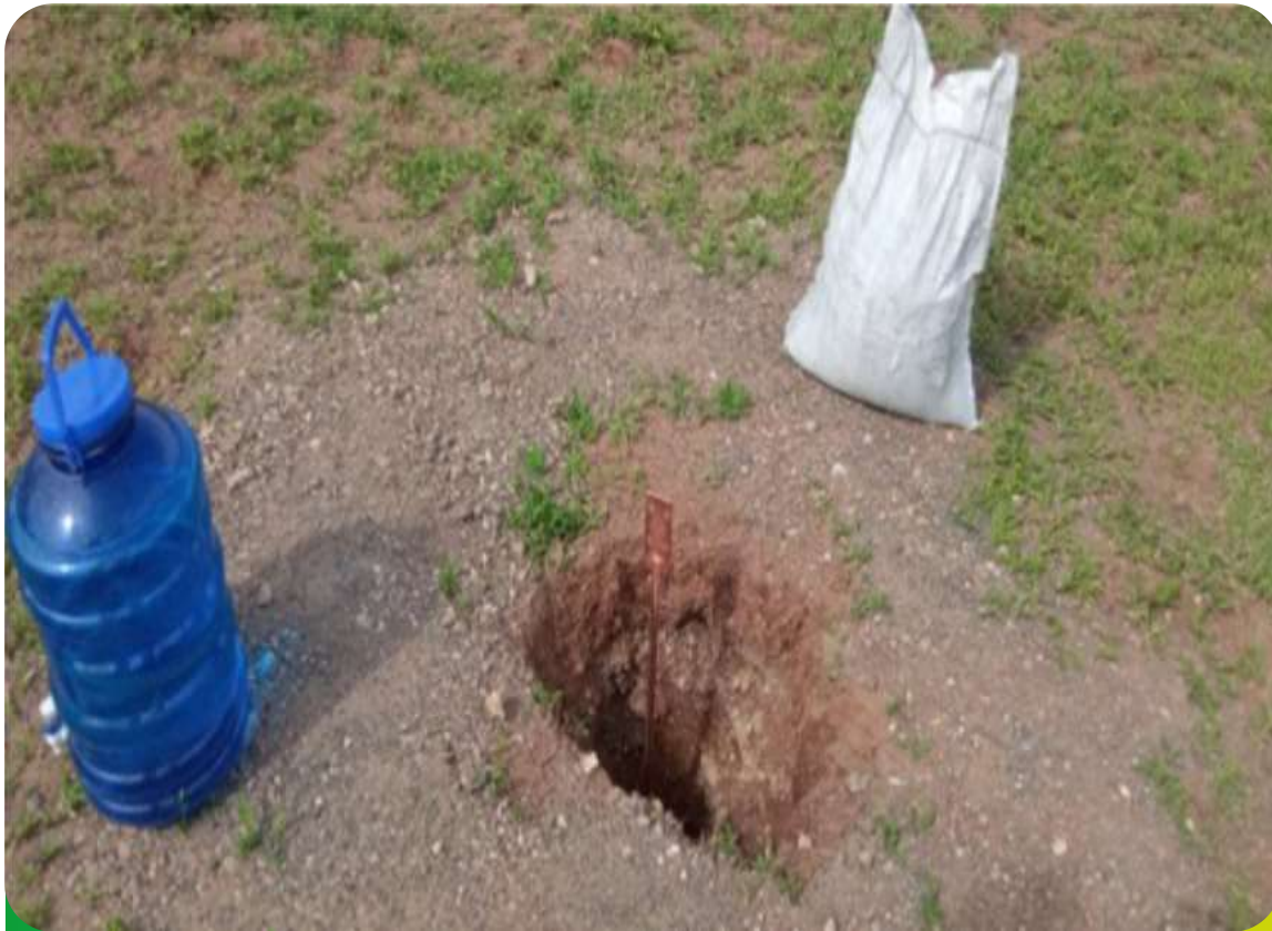
Earthing Rod Installation With
