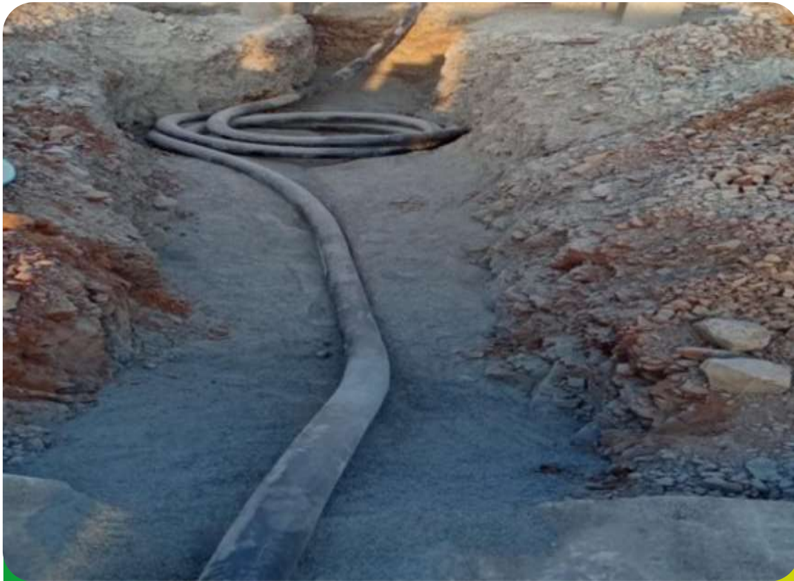
Cable Laying With Sand Bedding
