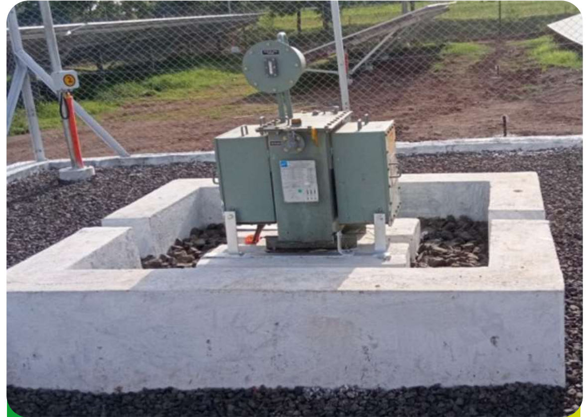
Auxiliary Transformer Foundation As Per Drawing
