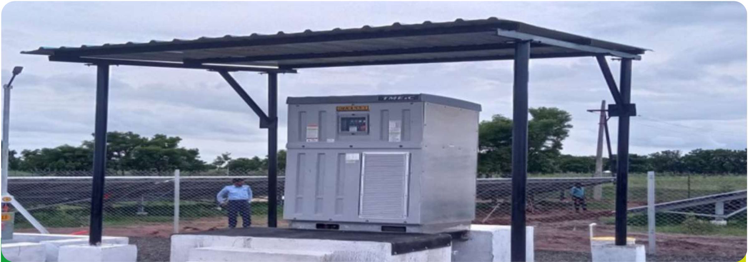
Inverter Foundation With Canopy Structure
