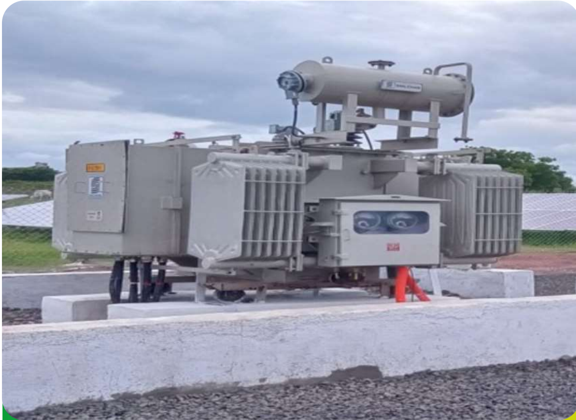
Main Transformer (idt) Foundation As Per Drawing
