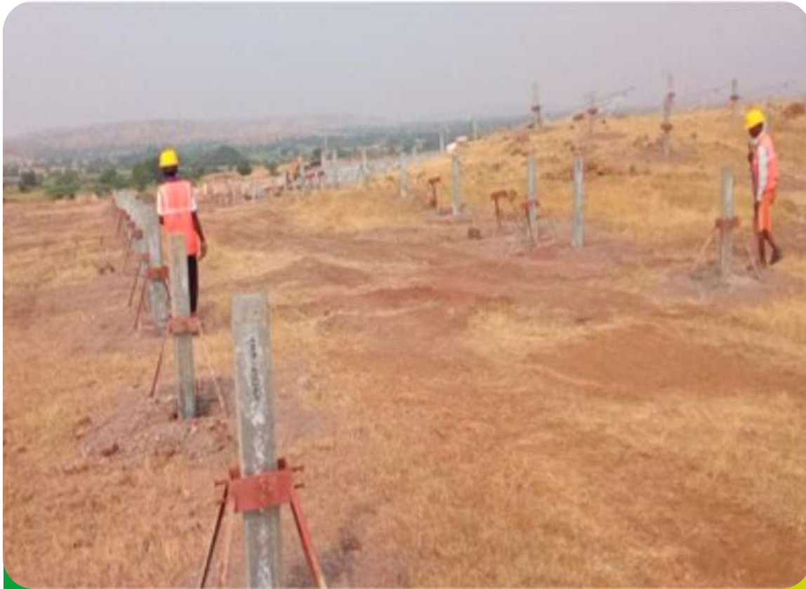
Pile Alignment And Curing
