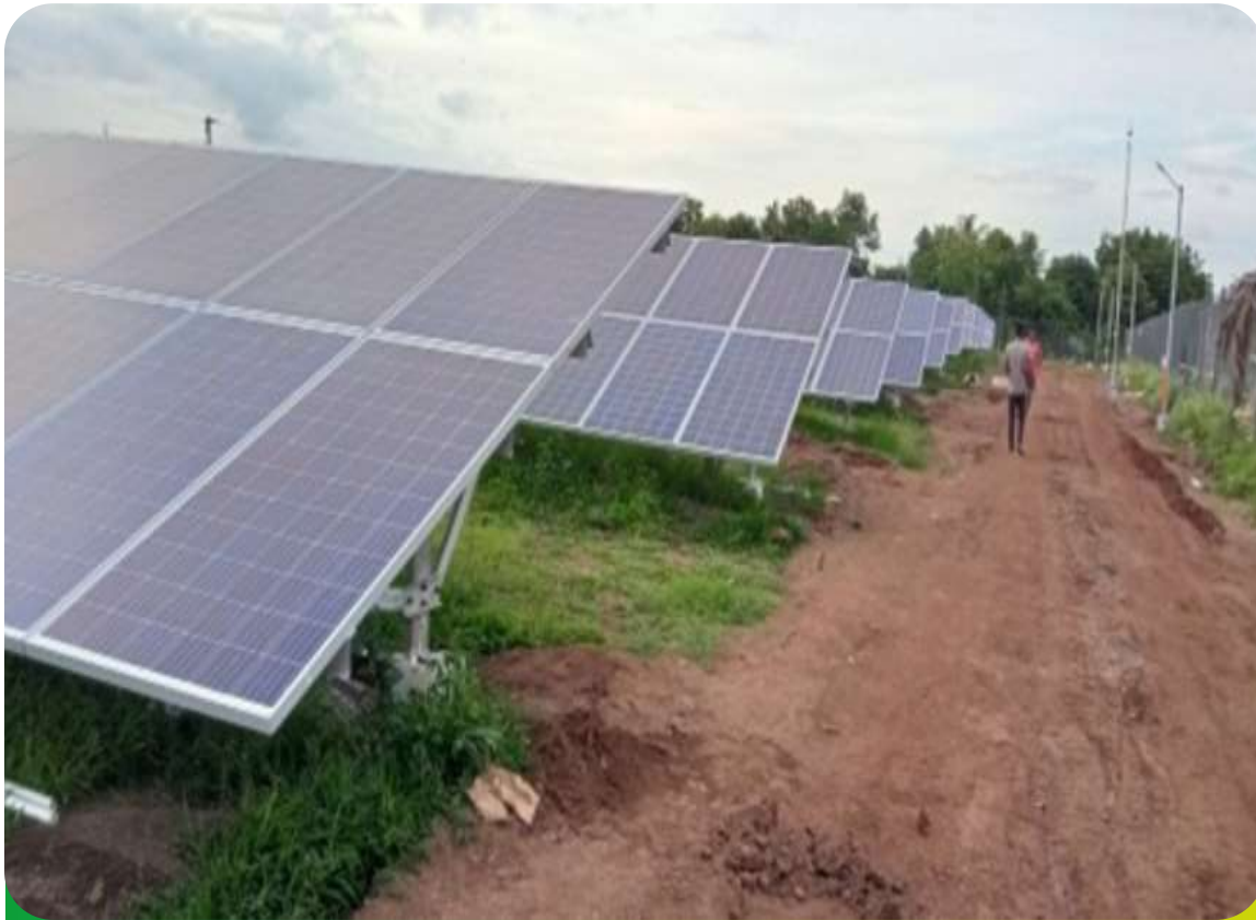
Proper Module Alignment With Tightening
