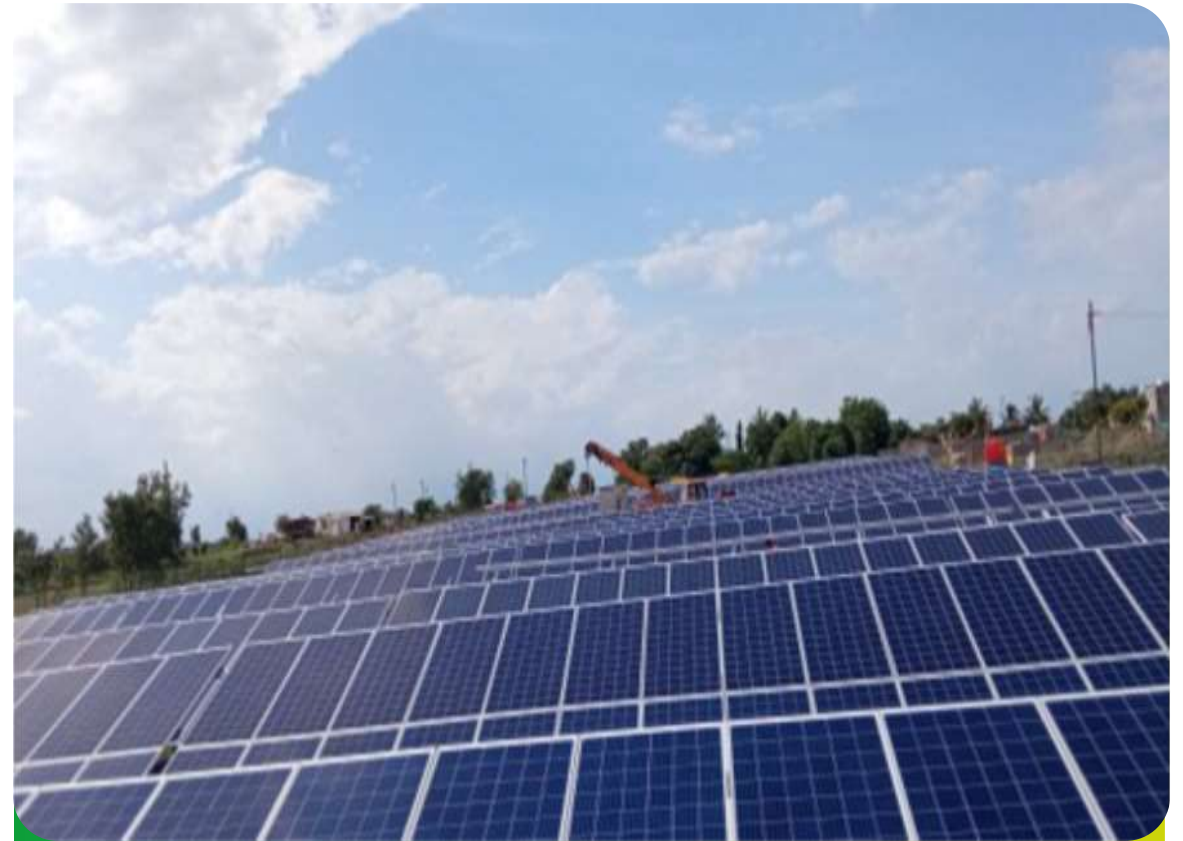
Proper Module Alignment With Tightening
